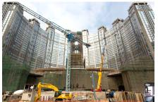
Studio City Macau is built on the reclaimed land of Cotai. Because of its proximity to the ocean a major concern was the chloride content of the high water table. Xypex was selected because of its proven track record for resistance to hydrostatic pressure and chloride attack. Xypex Admix was used to waterproof and protect over 100,000 m³ of concrete in the basement slab and walls.
